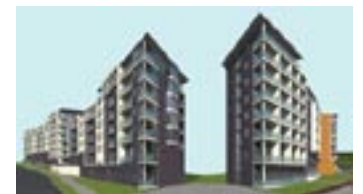
Image reproduced with kind permission of McCabe Builders
