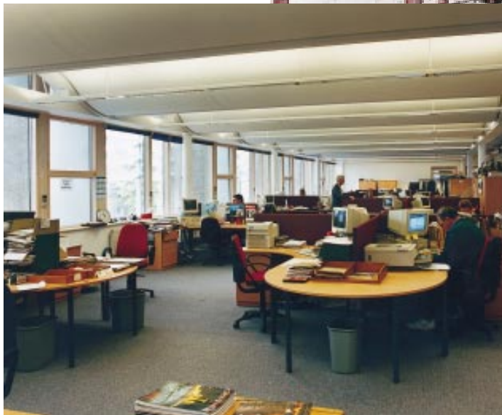
Above: Toyota's HQ in Epsom uses 'passive' exposed precast concrete soffit units throughout the office areas as part of a hybrid concrete frame. A precast floor unit being lowered onto falsework, Trent Concrete Ltd manufactured the precast columns and floor slabs.
