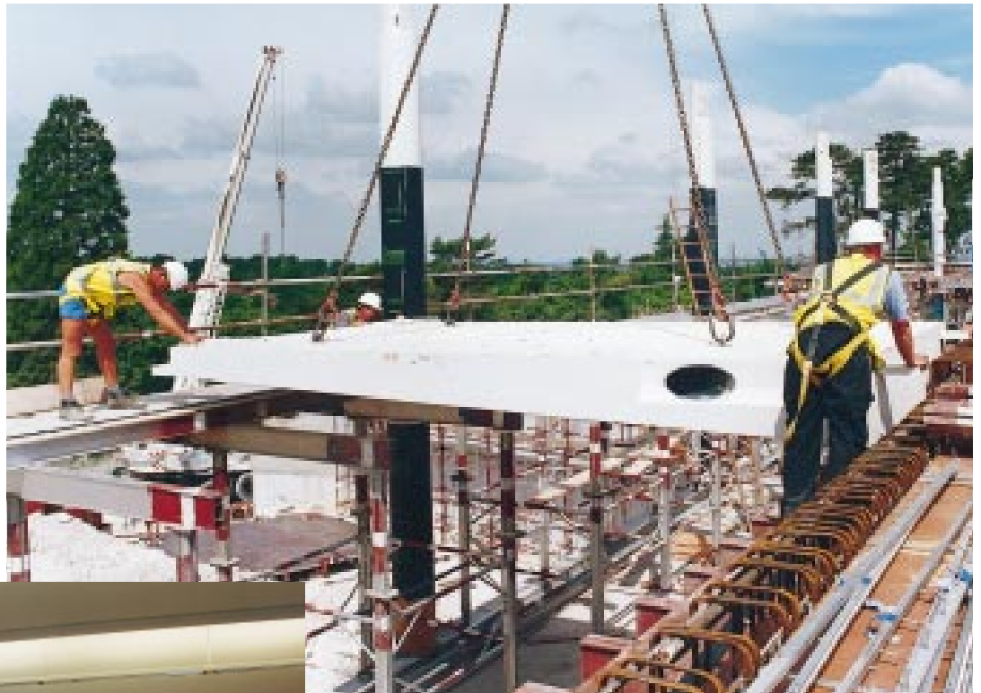
Above: Toyota's HQ in Epsom uses 'passive' exposed precast concrete soffit units throughout the office areas as part of a hybrid concrete frame. A precast floor unit being lowered onto falsework, Trent Concrete Ltd manufactured the precast columns and floor slabs.
