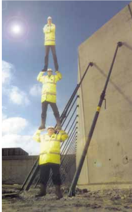
Standing on the shoulders of giants! RB Wonderwall – the tallest precast wall ever produced by top UK foundations expert Roger Bullivant Limited (RBL). Concrete Products national sales manager Trevor Howells is pictured in a "supporting" role with RBL's Paul Hayes and Gary Mills from Finnegan.
