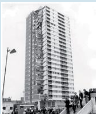
Photograph of the Ronan Point Collapse 1968.
